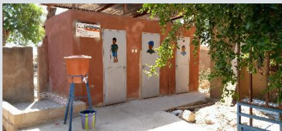
The new toilet block at Kokry HCF
