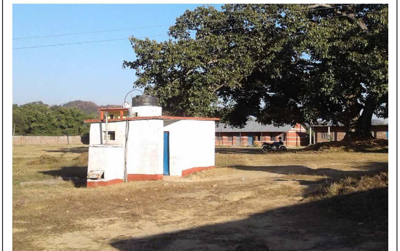
Fig 4: Gender friendly toilet with incinerator attached to the toilet for menstrual waste disposal
