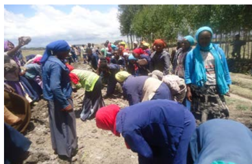
Community participation on trench excavation
